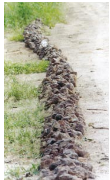
Saving the soil—building dykes to slow rain run off.
